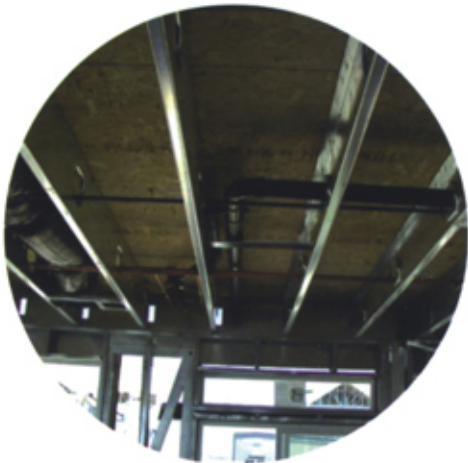
Facilities and lines hide in the stud
